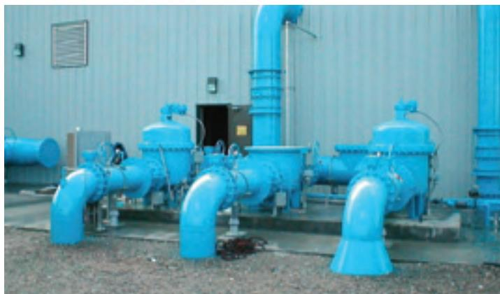
Eaton automatic strainers provide filtration of incoming water protecting membrane system in rigorous application including seasonal algae bloom.
