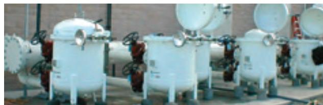
Eaton MAXILINE™ bag filter vessels. Pre-filtration of incoming well water protecting membranes in heavy metals abatement system for drinking water.
